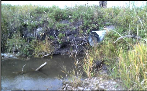
Erosion around a drainage inlet and sediment accumulation downstream of a washout
